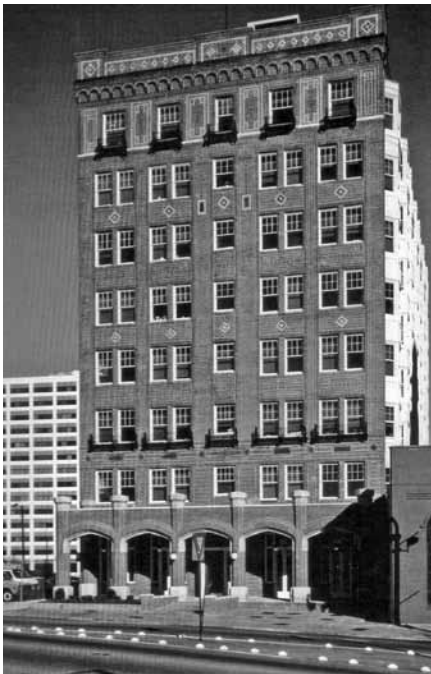
The front of The Imperial on Peachtree after the 1996 renovation of the Imperial Hotel. Photo courtesy of the Open Door Community via Gay Construction Co.
