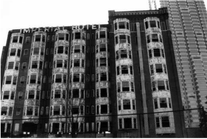
The side of the Imperial Hotel before completion of the 1996 renovation. Photo courtesy of Progressive Redevelopment.
