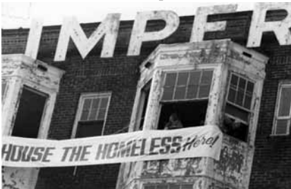
Photo courtesy of the Open Door Community.
